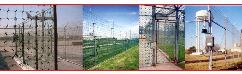
Any attempt to cut, lift, crawl under, or pass through the FiberNet will result in detection.
